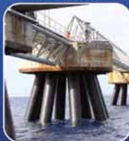
Steel & Concrete Pile Protection
