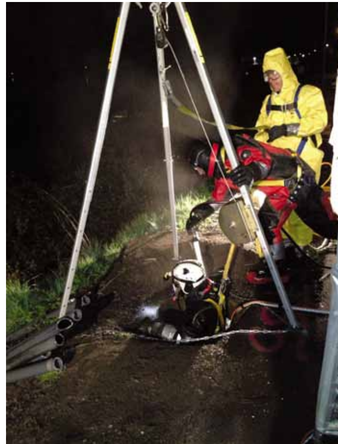
An Advanced Subsea Services diver enters the manhole.
