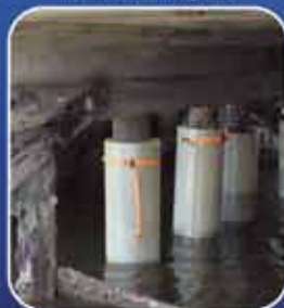
Timber Pile Structural Repairs
