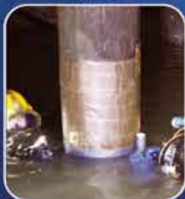
Timber Pile Protection
