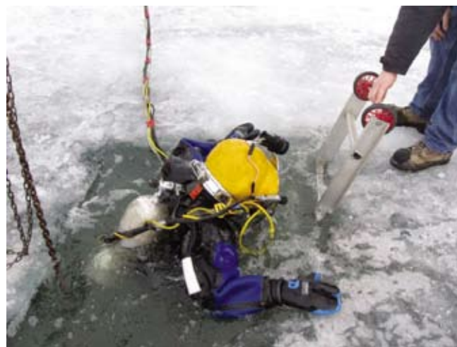
Diving through the ice on Lake Simcoe to complete repairs to outfall diffuser nozzles.
